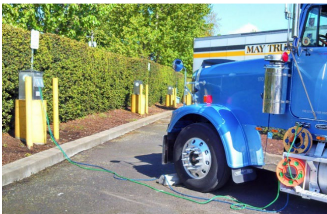
Figure 6.1 Truck Stop Electrification
